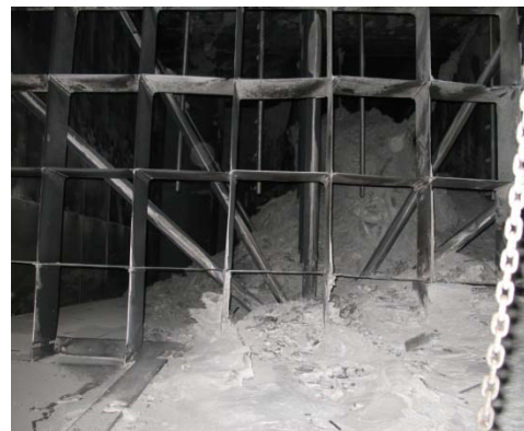
Inlet Turning Vane and Nozzle Pluggage
