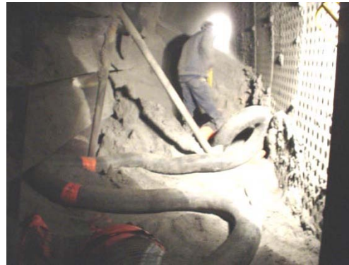
Inlet Turning Vane and Nozzle Pluggage
